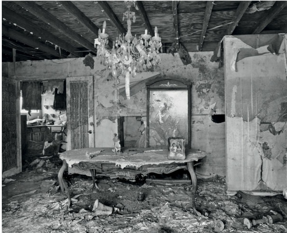
Abb. 18-4 Destroyed Home, Ninth Ward, New Orleans
